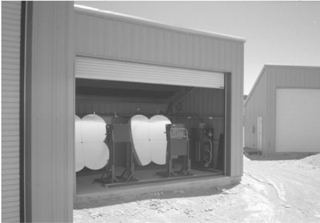
**Fig. 1.** Two detectors are housed in a single metal building. The large roll-up garage door opens for nocturnal observation. A door opened in daylight with the mirrors and clusters exposed is the researcher's worst nightmare.
